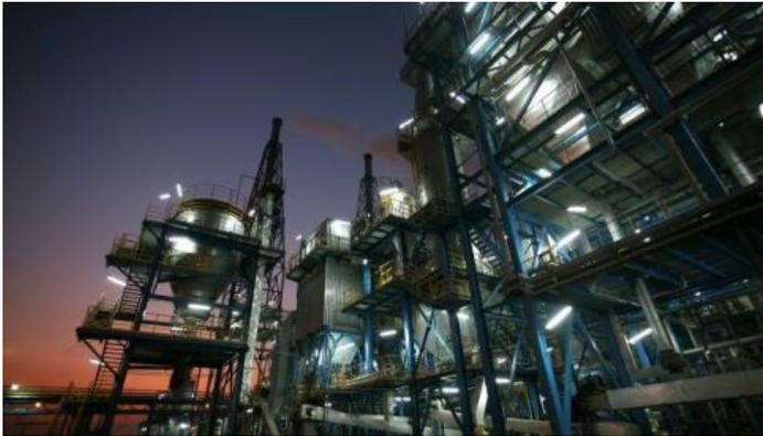
The facility is equipped with energy recovery devices. The heat generated by incineration is used to produce steam and supply to industrial companies in the park, reducing the consumption of fossil fuels, saving 55,000 tons of standard coal each year, maximizing the recycling of waste energy. It is also equipped with off-gas treatment system (removal of halogen, sulfur, heavy metals, dust) to strictly comply with the EU emission standard.
